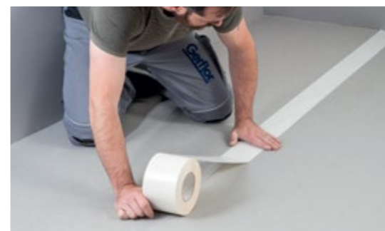
Place the HOP holding tape where the rolls join Code: 059E/Packaging: 50 ml/box
